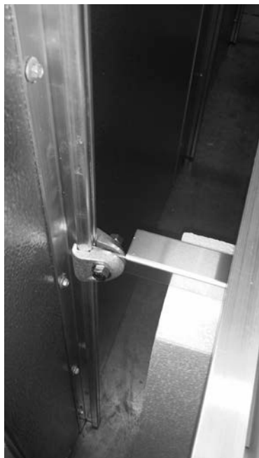
Figure 13: Cross braces attached to struts with clamps. See Figure 9 on pg 5.
