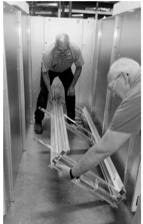
Figure 11: Telescoping tray inserted at a 45° angle.
